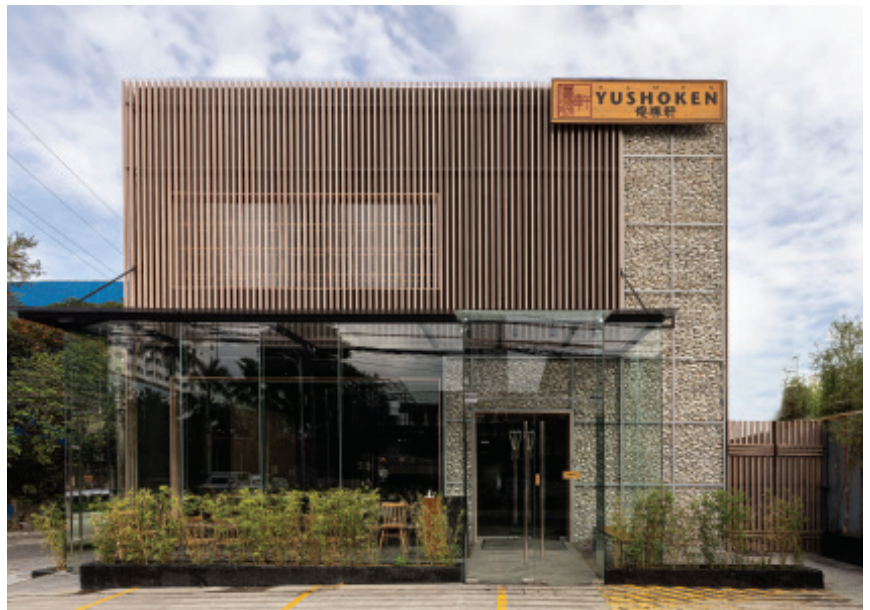
The contrast between the organic gabion walls and orderly wooden slats on Yushoken’s facade reflects the balance of natural and structured elements in Japanese design
